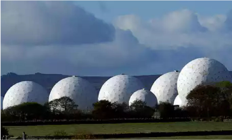
FIGURE 3 The radar domes of the RAF Menwith Hill facility in England 32
